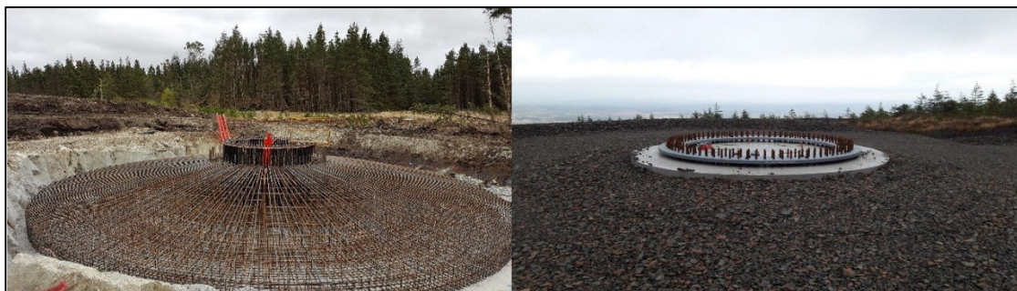
Plate 4-2 Turbine 'Anchor Cage' and finished turbine base
