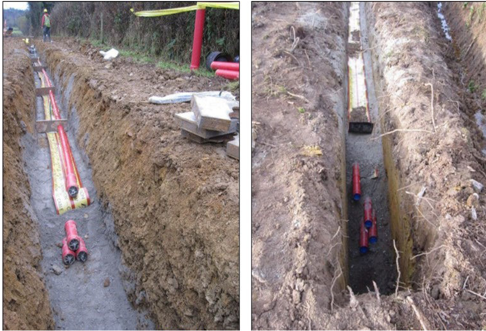
Plate 4-9 Typical Cable Trench View
