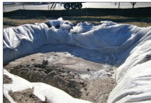
Plate 4-4 Concrete washout area
