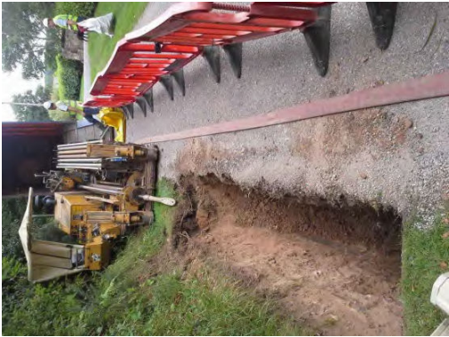
Typical Drilling Rig & Launch Pit
